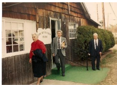
1 st Sims Mission building
